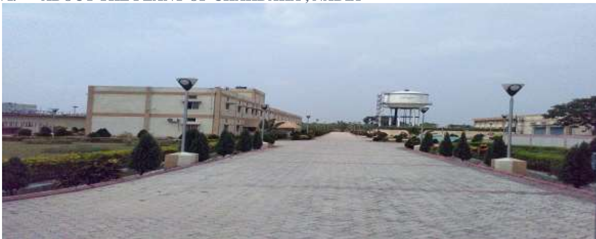
Fig: 4 Water Treatment Plant of Chakdaha
