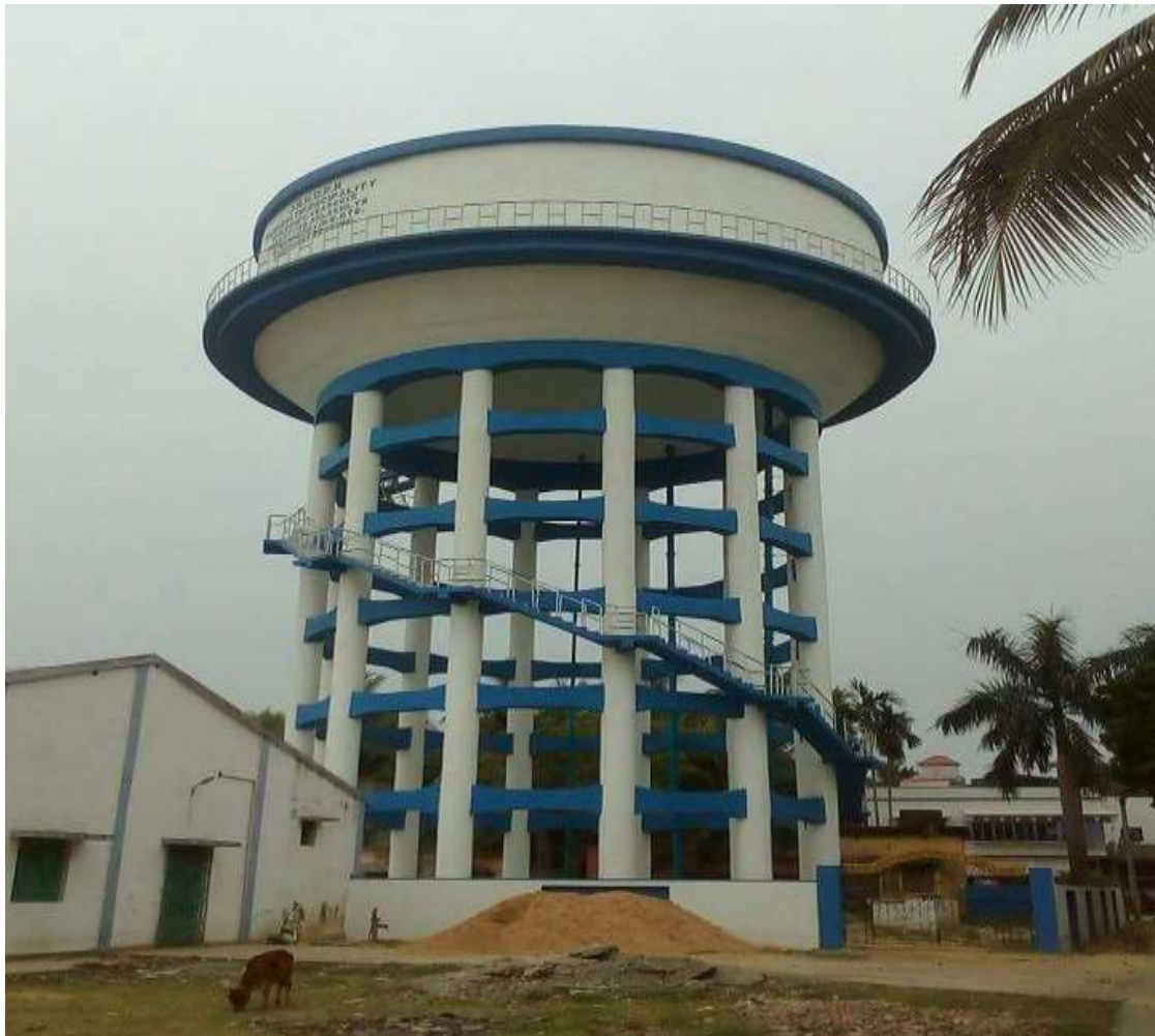
Fig : 6 Pump house and Storage Tank
